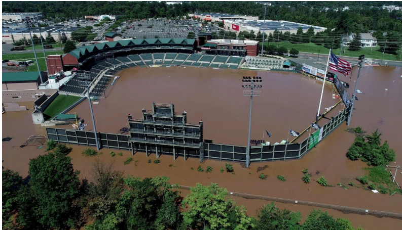
Figure 18: TD Bank Ballpark Flooded With Water Due to Hurricane Ida
